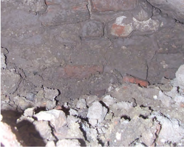
Figura 4. Foto interior pivnița P2 / Photo of the interior of cellar P2.
