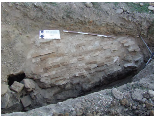
Figura 25. Foto extrados bolta B1 / Photo of the upper part of vault B1.
