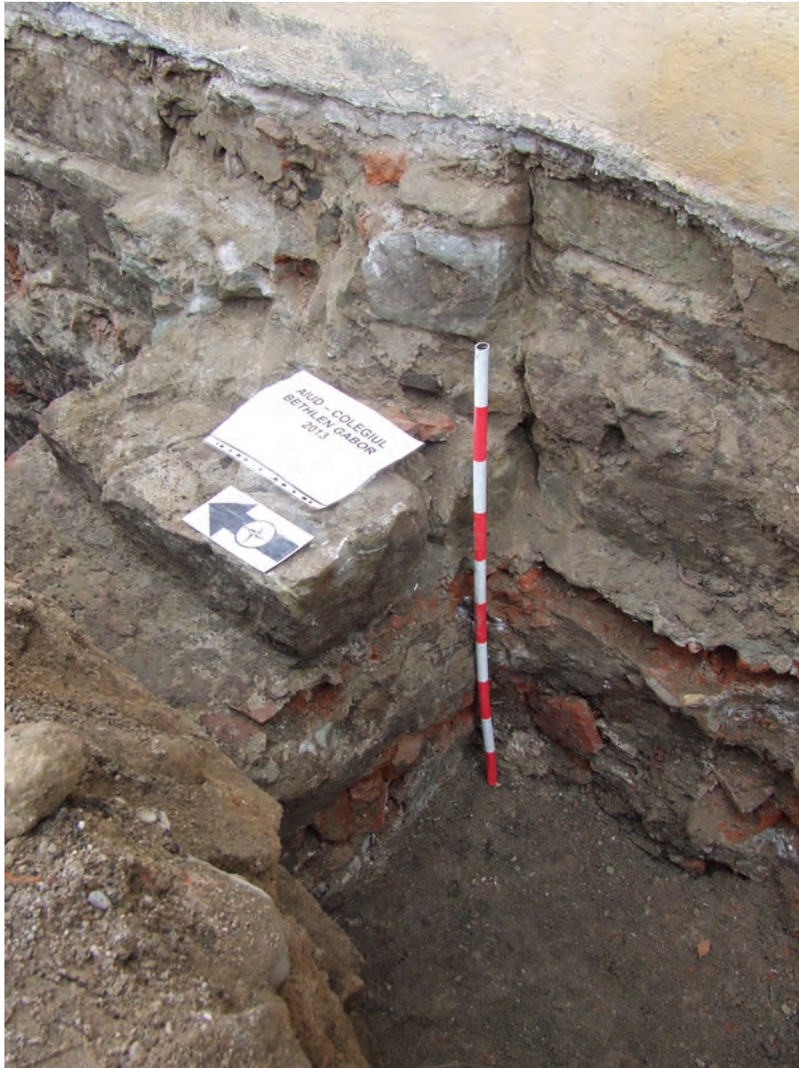
Figura 33. Latura de vest a corp C1, foto contrafort 1 / Western side of building C1, photo of counterfort 1.
